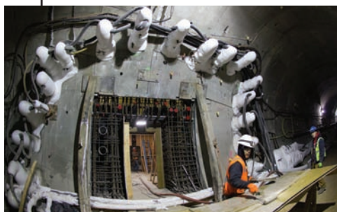
Left: A typical cross passage freeze to support excavation
