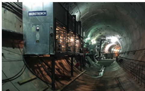
Left: A smaller refrigeration plant located in the tunnel
