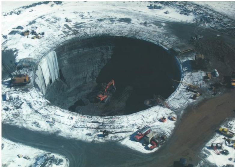
Figure 2. Excavation process of crown pillar
