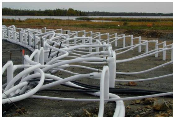
Figure 1. Freeze pipe configuration
