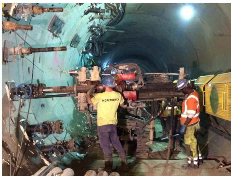
Horizontal Freeze Pipe Drilling
