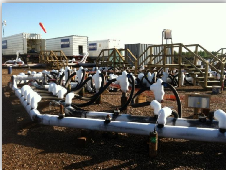
Freeze Coolant Distribution System
