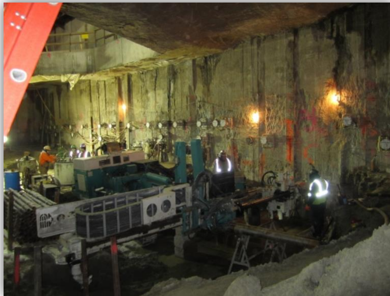
Horizontal Freeze Pipe Drilling
