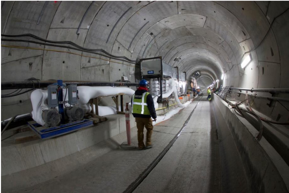
In-Tunnel Refrigeration System
