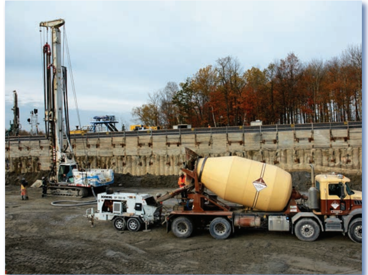
Pump transfers grout to RI tool.
