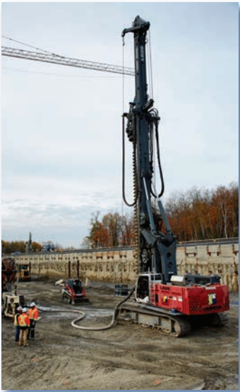
Above: Installing Rigid Inclusions for the construction of a train station.
