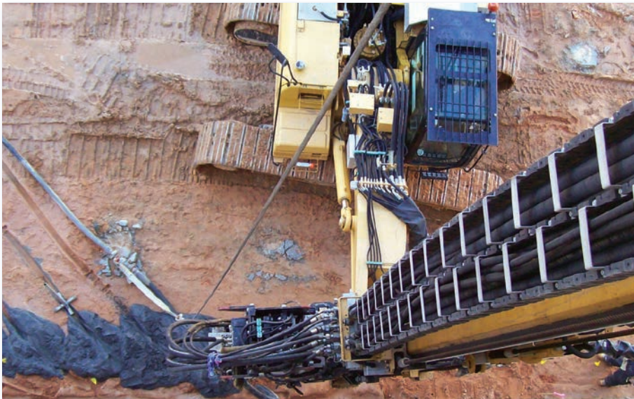
Rigid Inclusion installation for a planned hotel.
