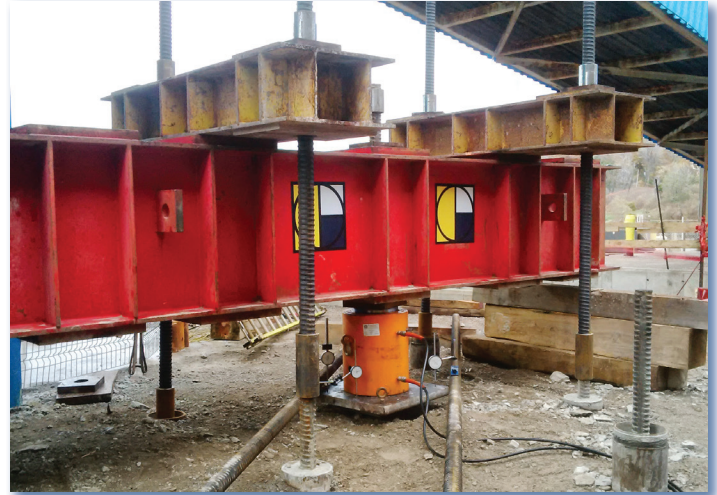
A compression load test being performed to 200% of design load.
