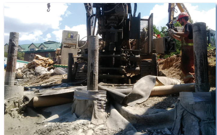
The composite structure of a micropile: outside casing, internal grout, and solid all-thread bar used for center reinforcement.
