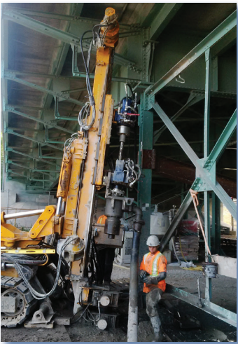
Above: Installation of micropiles for elevated highway with spoil control system.
