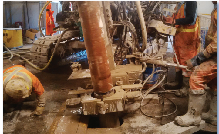
Casing installation for a large capacity micropile.
