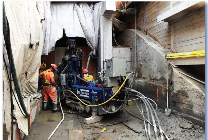
Low headroom jet grout rig.
