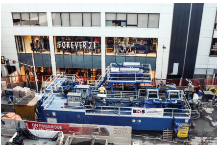
① Typical jet grout plant setup.
