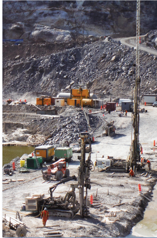
Jet grouting for seepage control.
