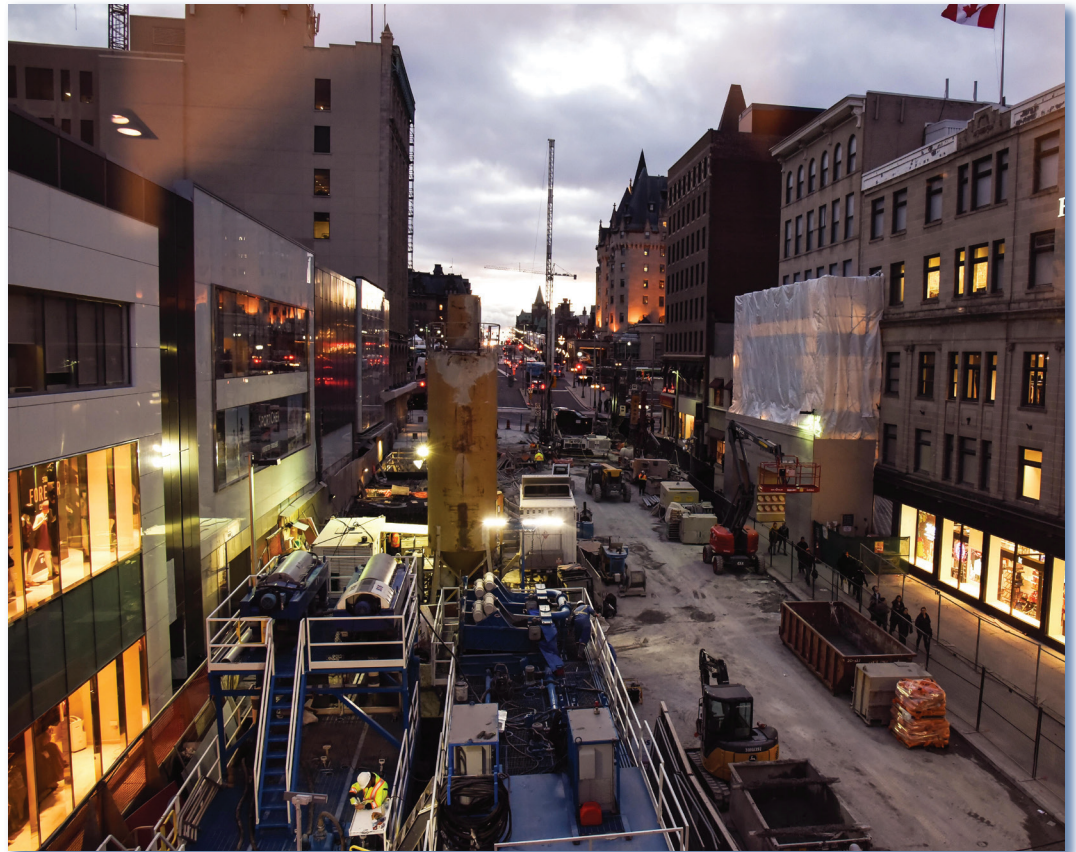
Above: Jet grout block for tunnel break-in/break-out.
