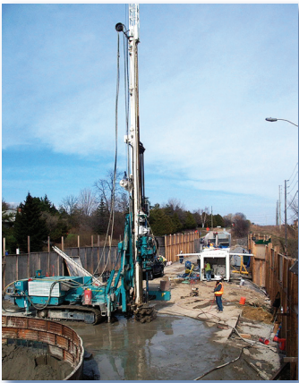
Above: Jet grout block for tunnel break-in/break-out.
