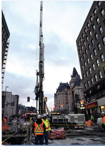
Jet grouting in an urban environment.
