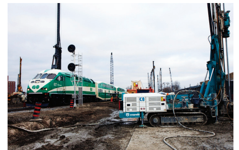
④ BOS system used to treat and separate spoils.
