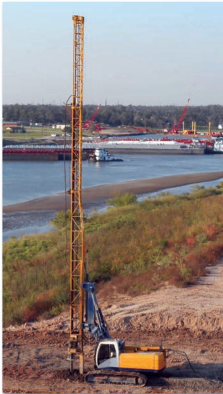
Dry soil mixing column rig and mast.
