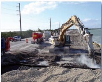
① Construction of a retaining wall for slope stabilization using dry soil mix columns.
