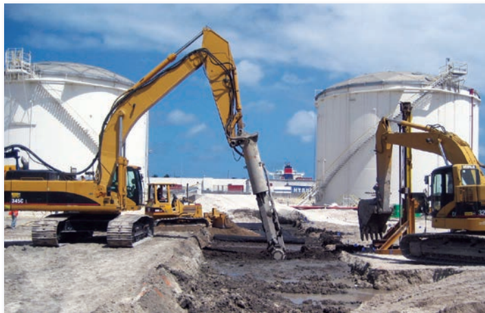
Mass mixing rig.
