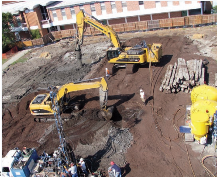
① Construction of a retaining wall for slope stabilization using dry soil mix columns.
