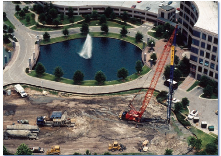
Compaction grouting to pre-treat the Summit site reduced the risk of future sinkhole activity.
