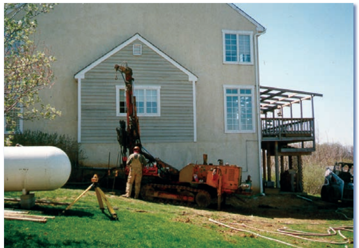
Compaction grouting was performed at interior and exterior locations, with minimal disturbance to townhouse residents.
