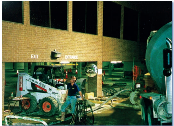
Compaction grouting stabilized the rubble fill underlying a four-story building and successfully restored the building to near original elevation.
