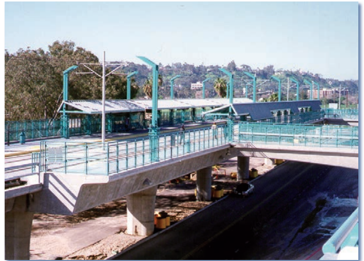
Pre-treatment with compaction grouting for long-term liquefaction mitigation protected the integrity of caissons supporting light rail piers.
