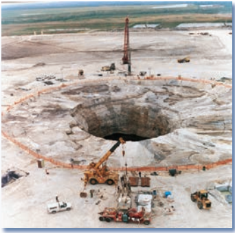
Compaction grouting was used to seal this 160-foot diameter sinkhole that extended down to the Floridan aquifer.
