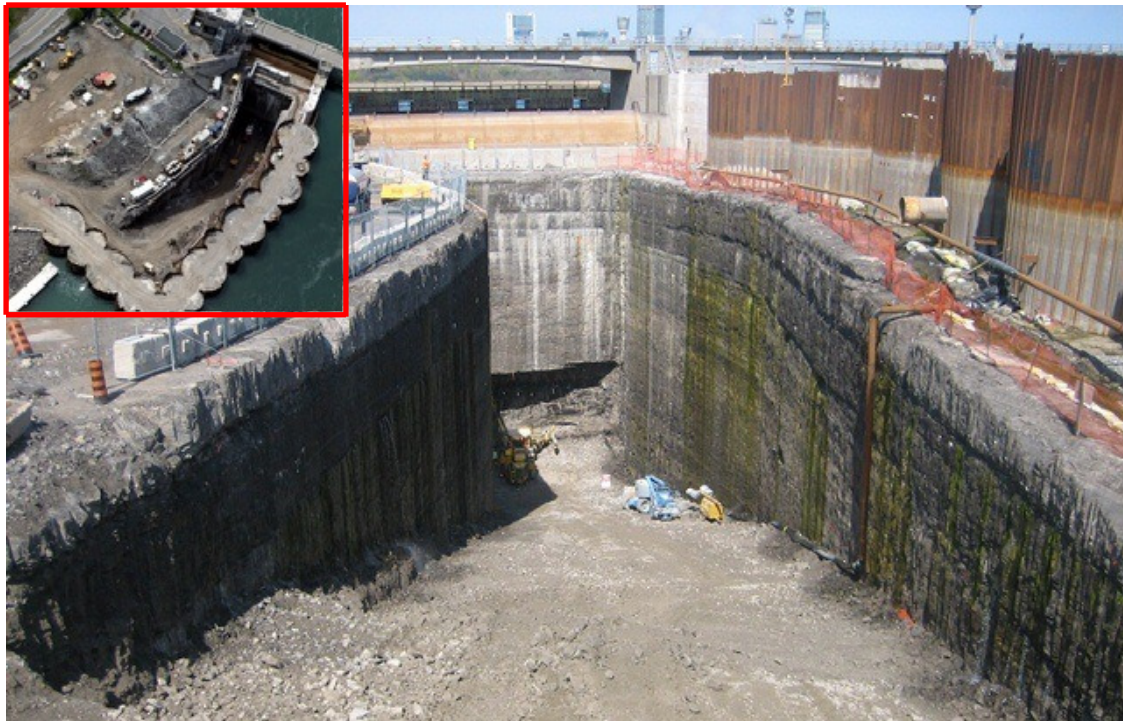
FIG. 6. Intake structure excavation
